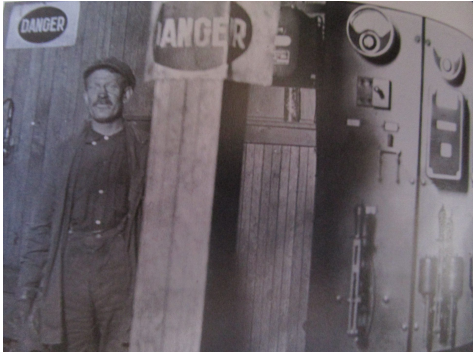
A worker poses next to an electrical switch panel inside the hoist house. This panel operated at 440 volts AC and controlled equipment above and below the mine.
