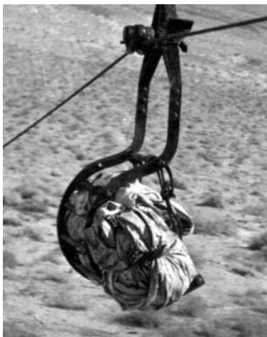
A similar carrier is used to transport bundled goods at the Keeler end of the tramway
