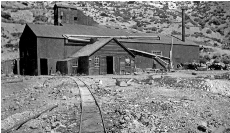
Tracks lead from the hoist house which houses the Belshaw shaft that extends 900 feet into the ground. The original structure was built during the silver and lead mining days of the 1870's as seen in this picture, before the Gordon expansion.
